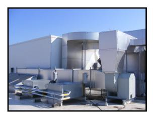
Eastern Industrial Services, Inc. is a certified installer\* of Techna-Duc®, a patented premanufactured insulating panel system. The unit is manufactured as a four panel system, constructed of Dow Thermax Polyisocyanurate Insulation. The insulation is laminated in a two inch thick, multilayer
