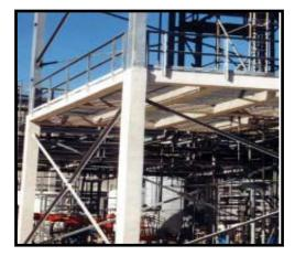
For new construction, Eastern Industrial Services, Inc. offers shop applied fireproofing, field applied fireproofing, or both. Structural steel members and equipment supports can be partially fireproofed at our shop, leaving the field connections bare. The field connections are fireproofed at the jobsite after erection. This combination offers significant cost savings and less manpower required to complete the work after erection, reducing congestion at the jobsite.
